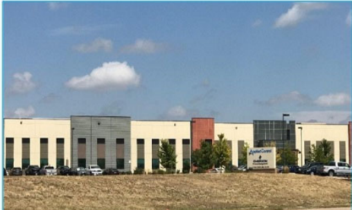
Applied Control Equipment – Denver, CO
